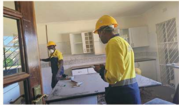
KITCHEN WORK IN PROGRESS
