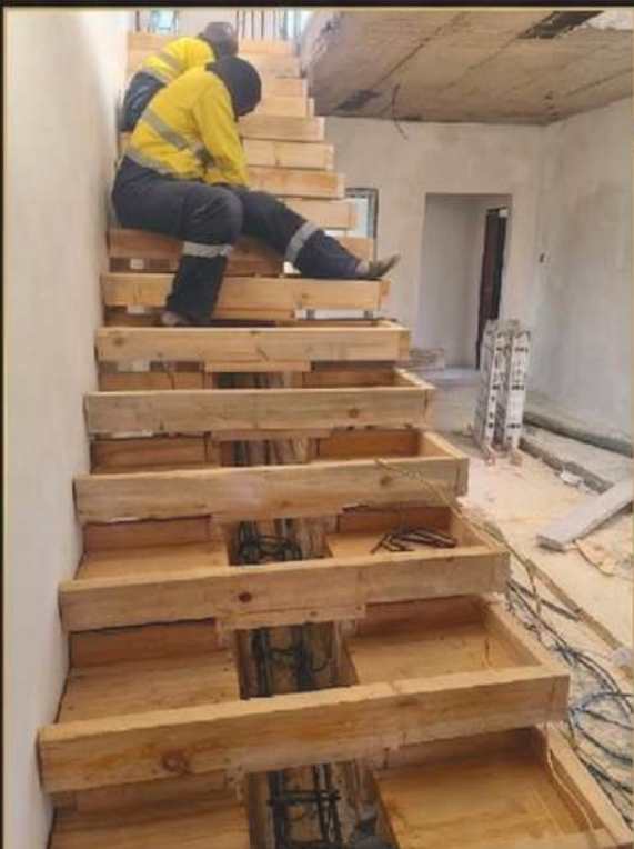
Structural Framing
